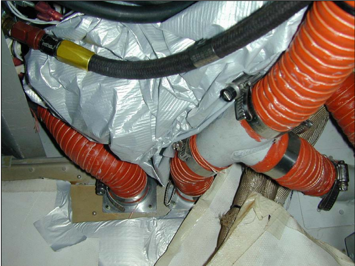
Figure 6: Completed LHS modification viewed from inside the aircraft.
